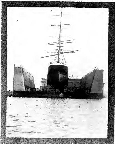
The Chilean bark "Llanquihue," the first sailing vessels to be taken out of the water by the new Todd Drydock at Tacoma. The new dock is operating very successfully.
